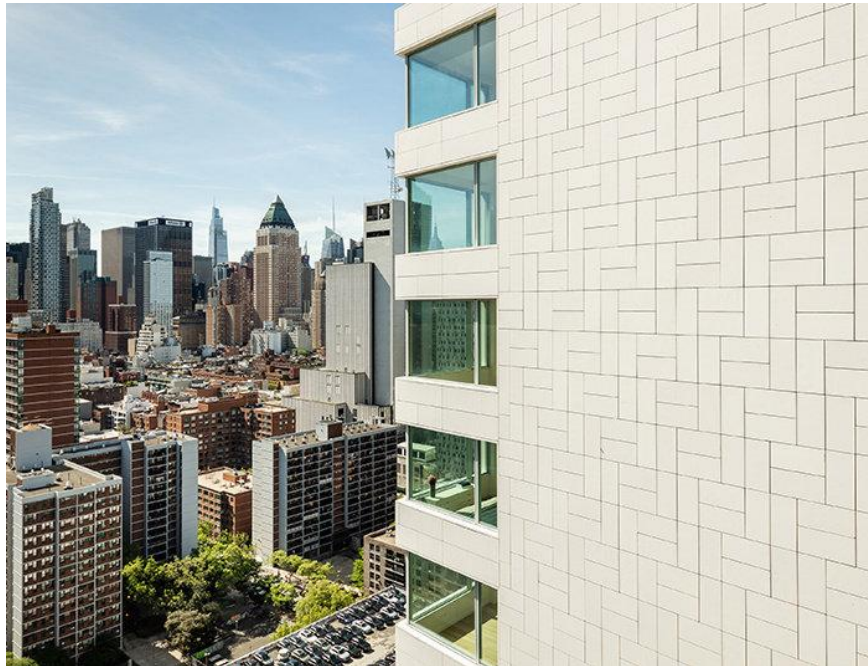
Corner windows lighten the mass of the building while maximizing the views of the city from inside
